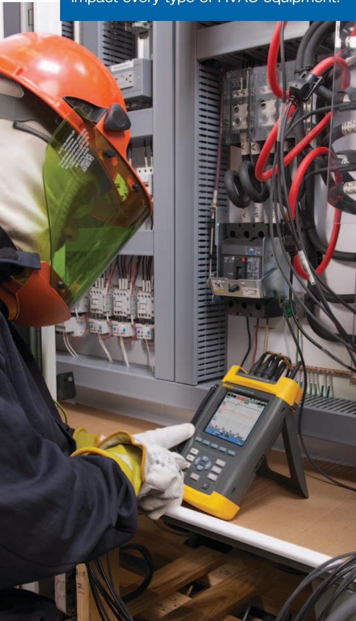
A technician recently documented the fault codes received when a chiller circuit tripped. A close look at the chiller revealed that the indicated faults did not match up to what was going on with the unit. Diagnostics indicated the chiller had undergone a “phase reversal” and, some time later, a “compressor motor overload.” Also, a “condenser pump variable speed drive fault” warning had been received.
